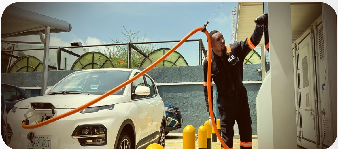
Figure 3: A technical staff of Folti monitoring the charging operation.
